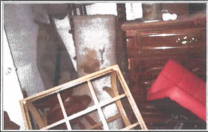
Unit 11 being renovated
