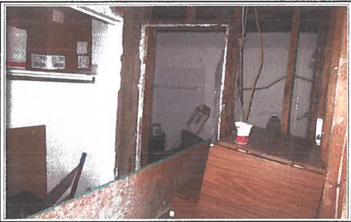
Unit 11 being renovated
