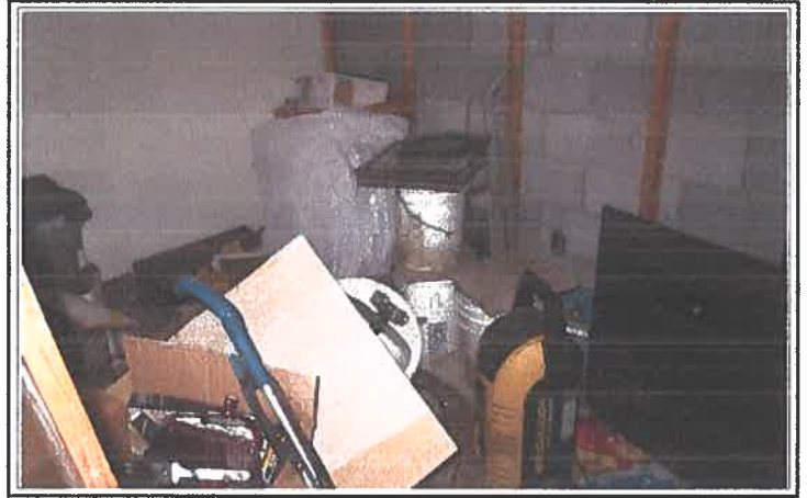
Unit 11 being renovated
