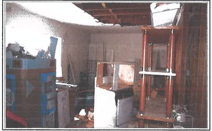
Unit 11 being renovated
