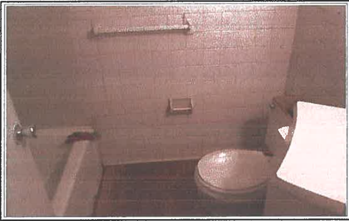
Bathroom, alternative view Unit 7
